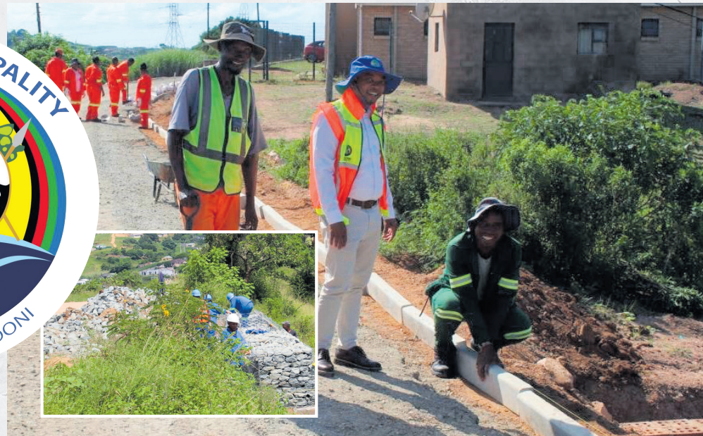
Installation of kerbs taking place on Mafithini Road in Ward 9. Inset: Installation of gabions designed to reinforce road infrastructure that is being upgraded.
